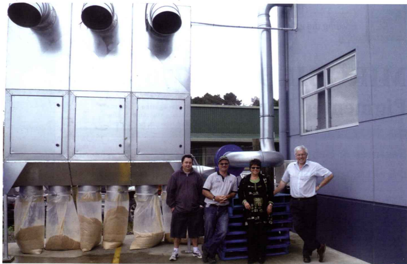
Michael McCartain factory manager, owners Mike and Kerri Lewin and Geoff Ebdon from NZ Duct&Flex next to the modular filter installed in September.
